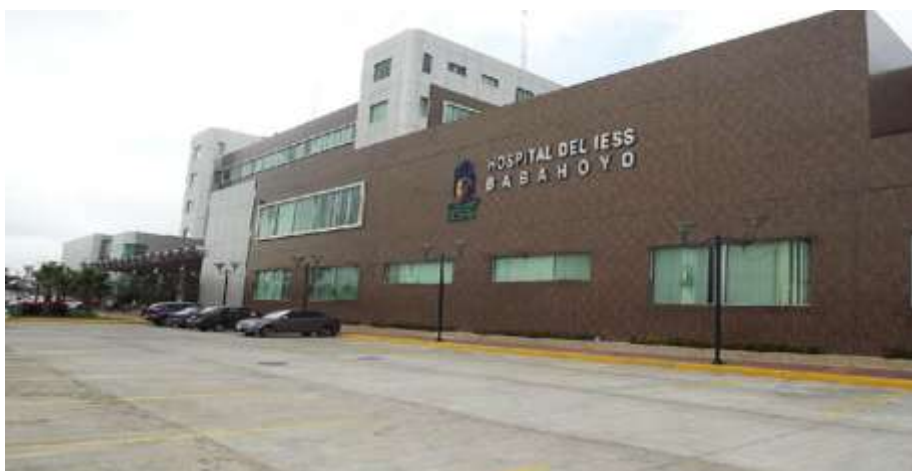
Figura 1: Hospital IESS BABAHOYO
